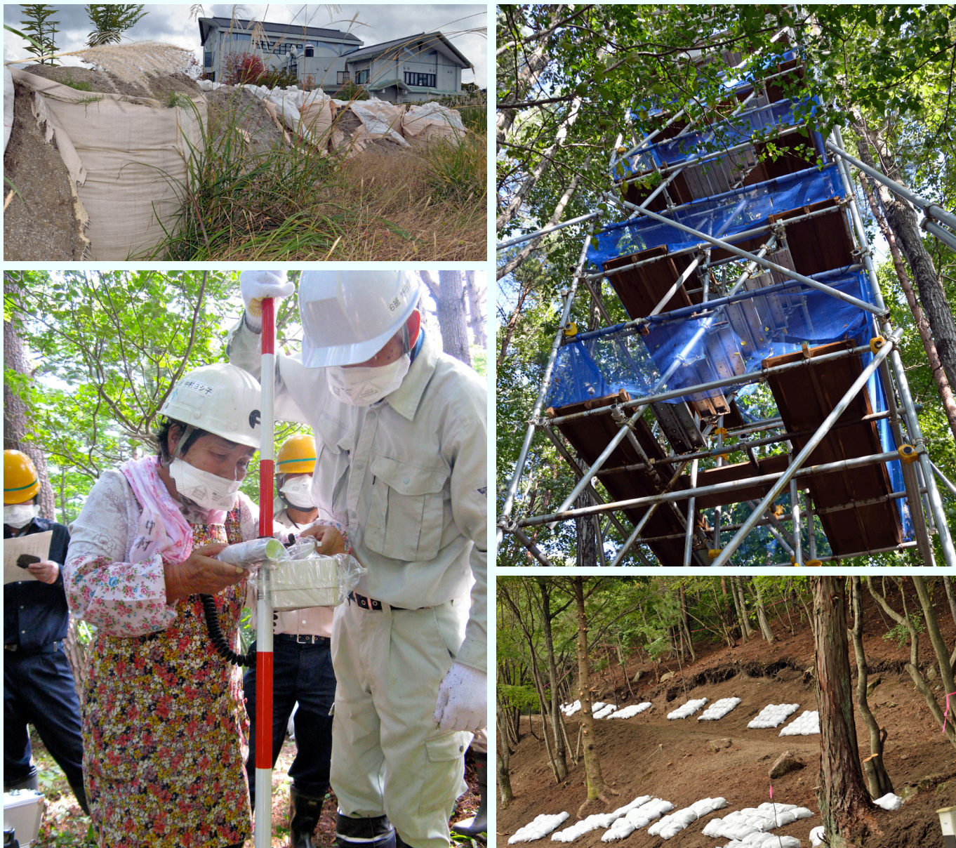
Clockwise from top left: Bags of contaminated soil from Iitate; a tower for monitoring movement of radionuclides in Kawamata; trial decontamination behind a home in Kawauchi; forestry and construction workers join in forest decontamination training at Forest Park Adatara, Otama.
